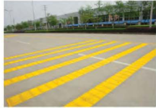
Road Marking Removal
