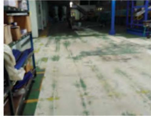
Old Epoxies Removal
