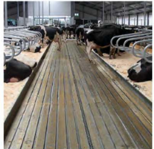
Farm Yard Floor Groove Cutting
